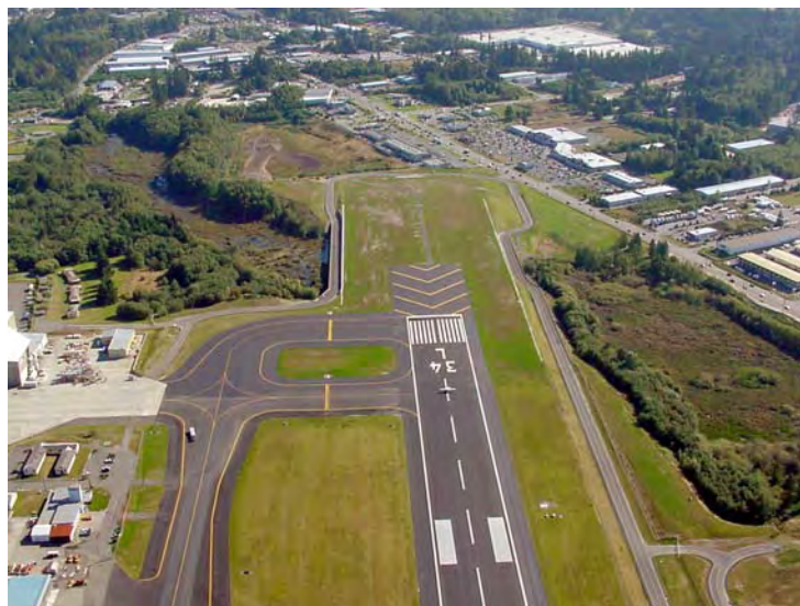
Paine Field Runway Safety Area Project completed in October 2001
