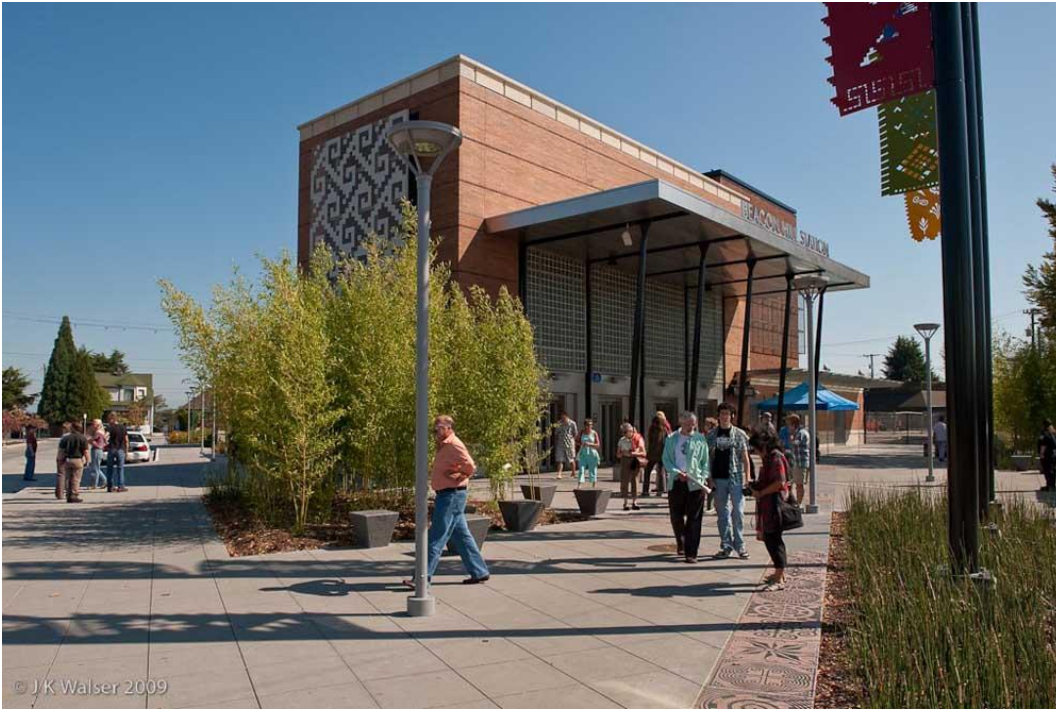
Beacon Hill Station
