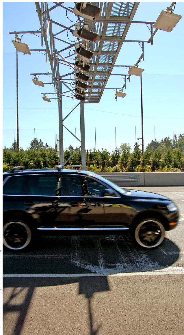
Tacoma Narrows Bridge electronic tolling, WSDOT
