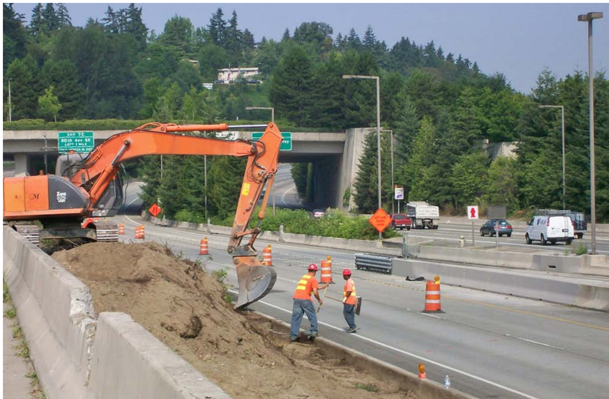
I-90 Two-Way Transit & HOV Operations Project, Mercer Island, WSDOT
