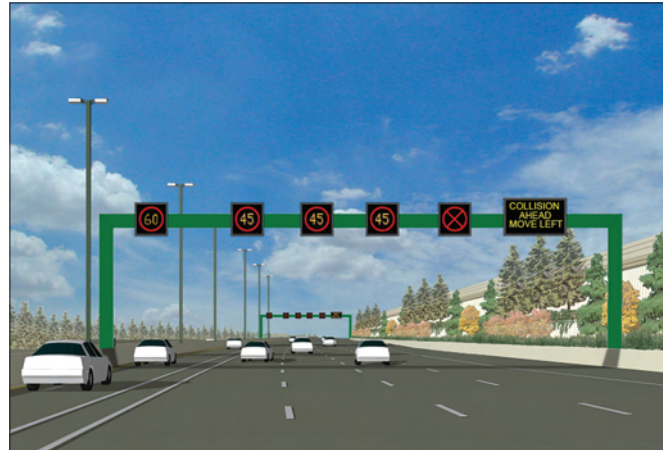
Example of speed harmonization and queue warning system as part of the I-405 Corridor Program roadway expansion.
