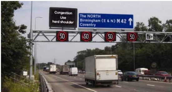
A gantry with dynamic lane speed on England's M42.
