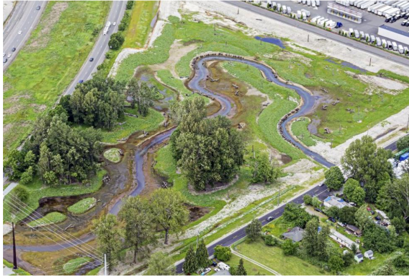
Wapato Creek Habitat Project
