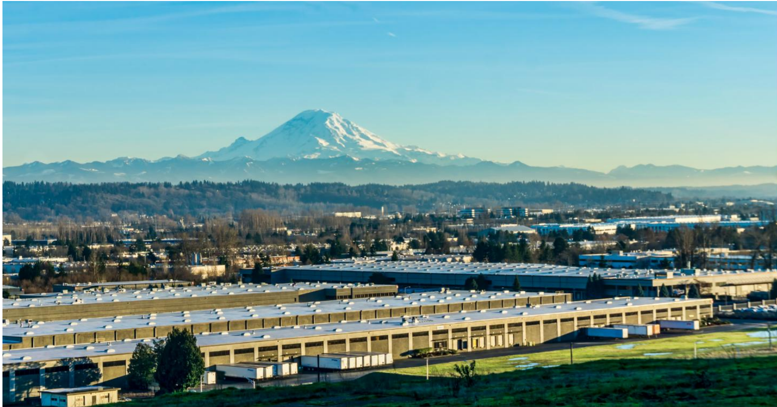
Kent Valley Industrial Center
