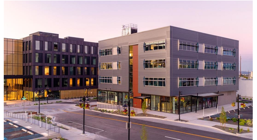
At South Landing Ecodistrict in Spokane, WA, buildings share energy through a micro-transactive grid, which minimizes impact on the City's power grid and creates a local energy market. Source: Catalyst Spokane.
