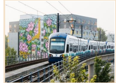
Mercy Housing Gardner House
