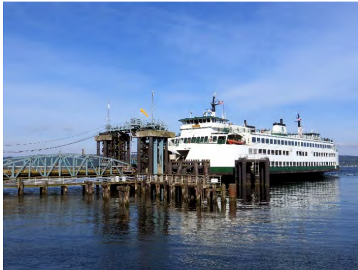
Mukilteo Ferry Dock
