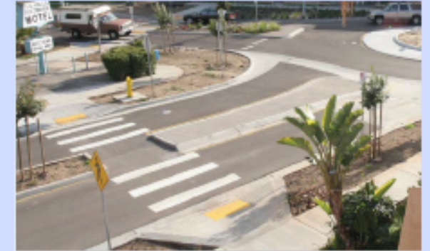
Median and pedestrian crossing islands near a roundabout.
