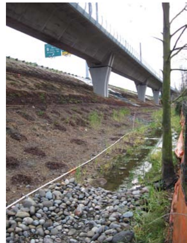
Sound Transit's light rail service from Sea-Tac Airport to downtown Seattle started operation in 2009.
