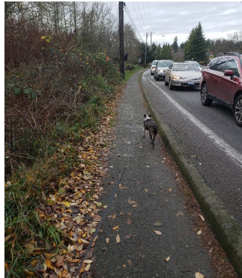
Phase 3 – Narrow, informal 2' wide asphalt path adjacent to 196 th Street SW; looking east and west.
