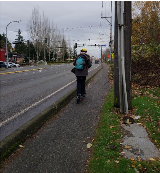
Phase 3 – Narrow, informal 2' wide asphalt path adjacent to 196 th Street SW; looking east and west.
