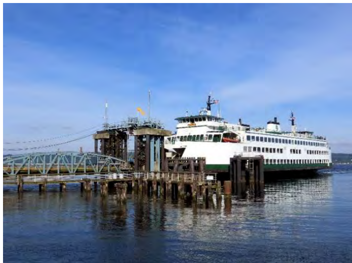
Mukilteo Ferry Dock
