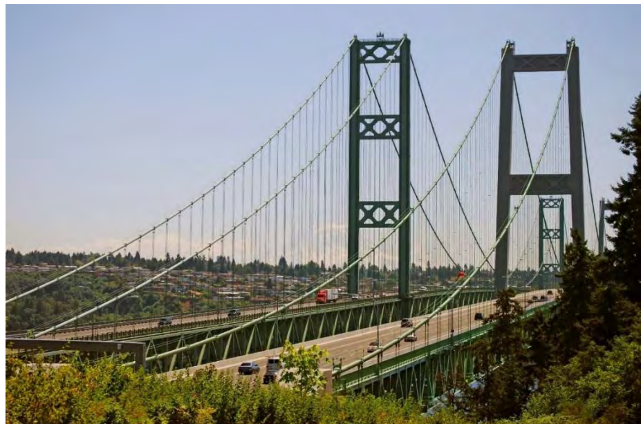
Tacoma Narrows Bridge
