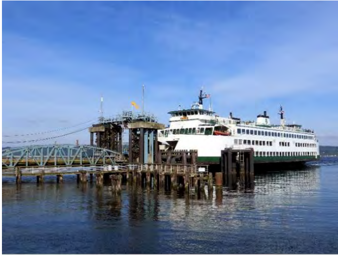
Mukilteo Ferry Dock
