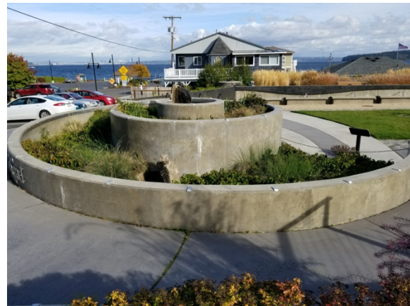
Manchester Stormwater Park in Kitsap County
